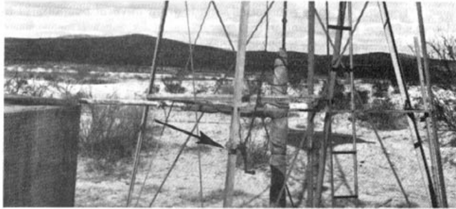
Windmill. Note windlass (arrow).
