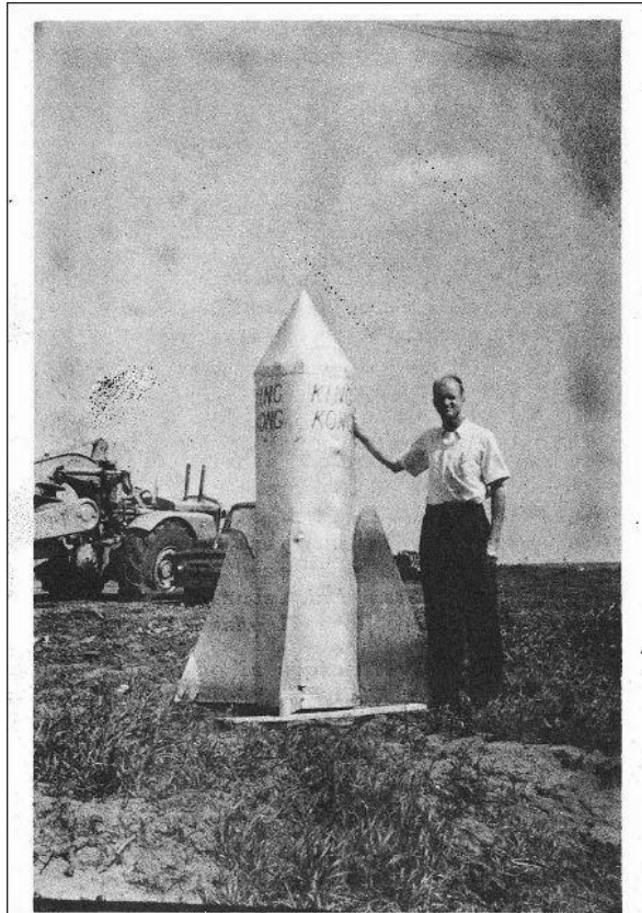
Walter Gormley and KING KONG set up on Site C
