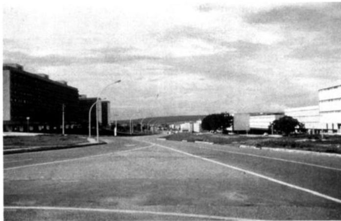
20. Residential access way L1 in Brasília, 1980
