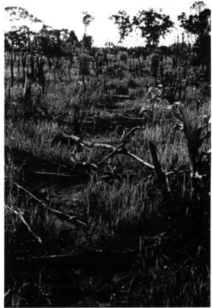
35. Construction of stick bunds across incipient gullies in a Sierra Leone rice field
