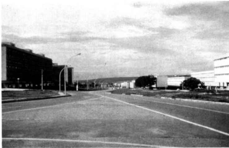
20. Residential access way L1 in Brasília, 1980
